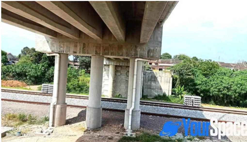
Ktmb buloh kasap feeder station 132 25kv buloh kasap
